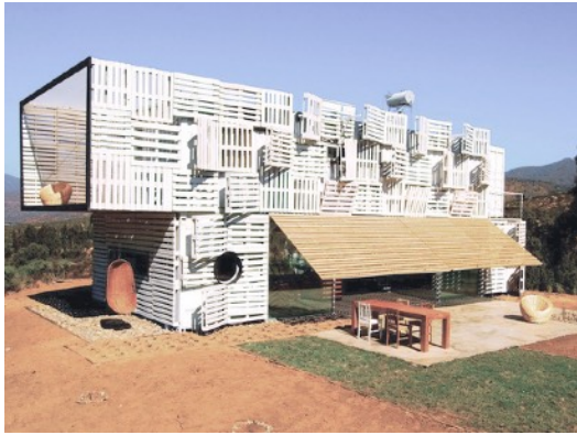
James et Mau Architects, Infiniski House, 2009
